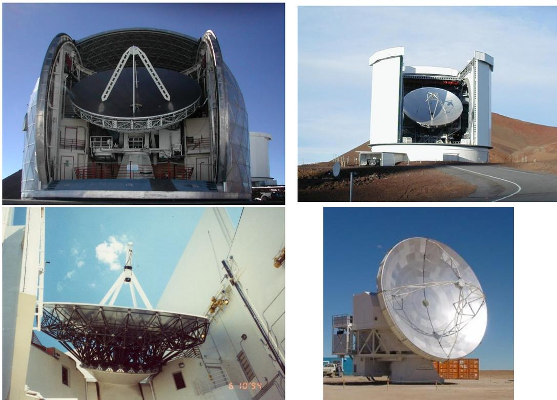
Slide 14. Submillimeter telescopes; from top left clockwise: CSO-10.4 m-Hawaii-1986, JCMT-15 m-Hawaii-1987, APEX-12 m-Chajnantor-2005, HHT-10 m-Arizona-1994.
