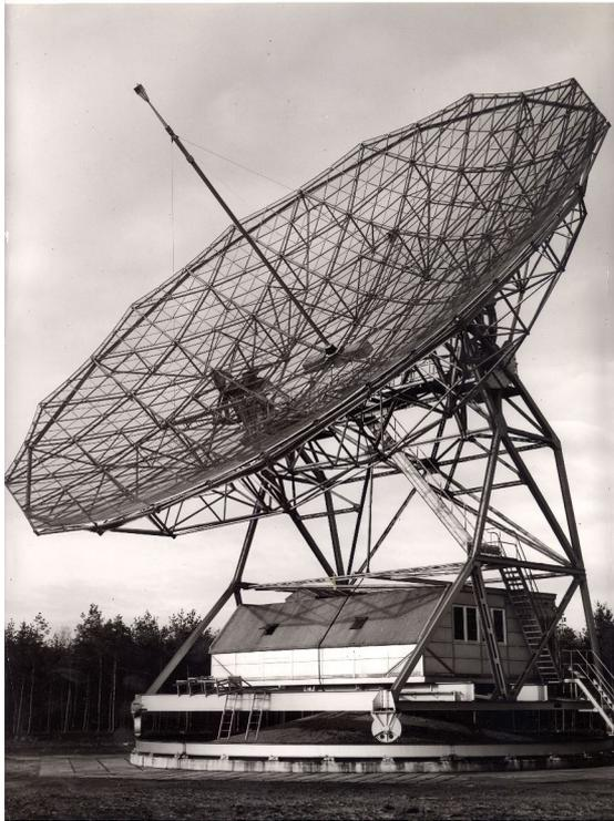
The telescope uses the primary focus with a central mast supporting the detector. A truss-frame supports the reflector with a rather large  $f/D=0.5$  that allows for flat triangular surface panels. The reflector is attached to the elevation bearings at about two-thirds of the radius. The alidade is a wheel-on-track system.
