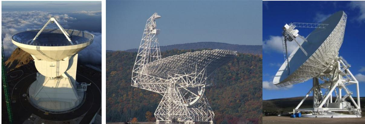
Slide 16. LMT-50 m-70  $\mu\text{m}$  surface in Mexico; GBT-105 m-400  $\mu\text{m}$  in the USA; SRT-64 m- 300  $\mu\text{m}$  in Sardinia, Italy. All use tilt meters for pointing correction and thermal sensors for surface correction.
