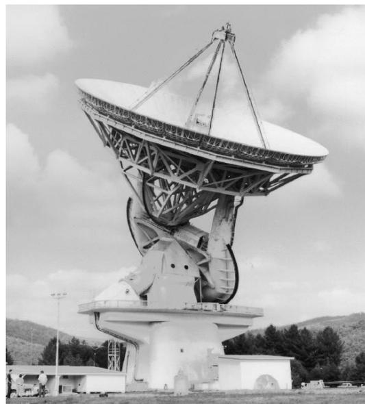
Slide 8. Equatorial mounts of the NRAO 85-ft “Howard Tatel” telescope (1959) with large gear-racks and the 140-ft (1965) with hydrostatic bearings and aluminium backup structure.
