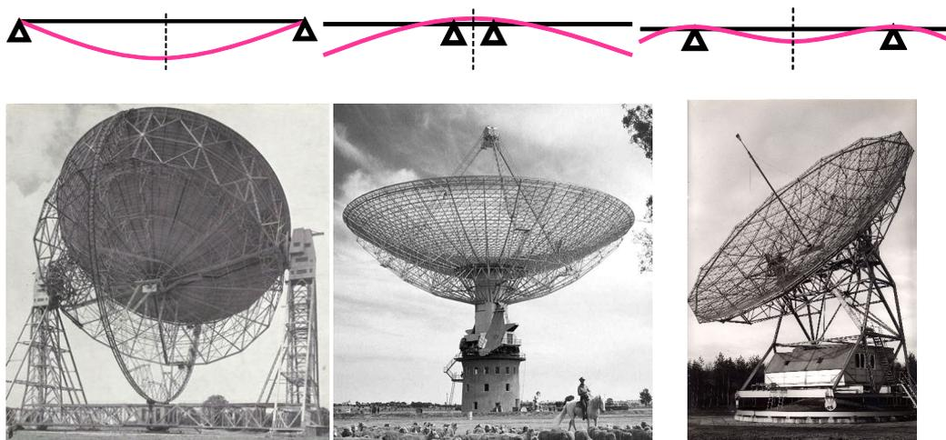
Slide 7. The deformation pattern dependence on location of connection to elevate bearings.
