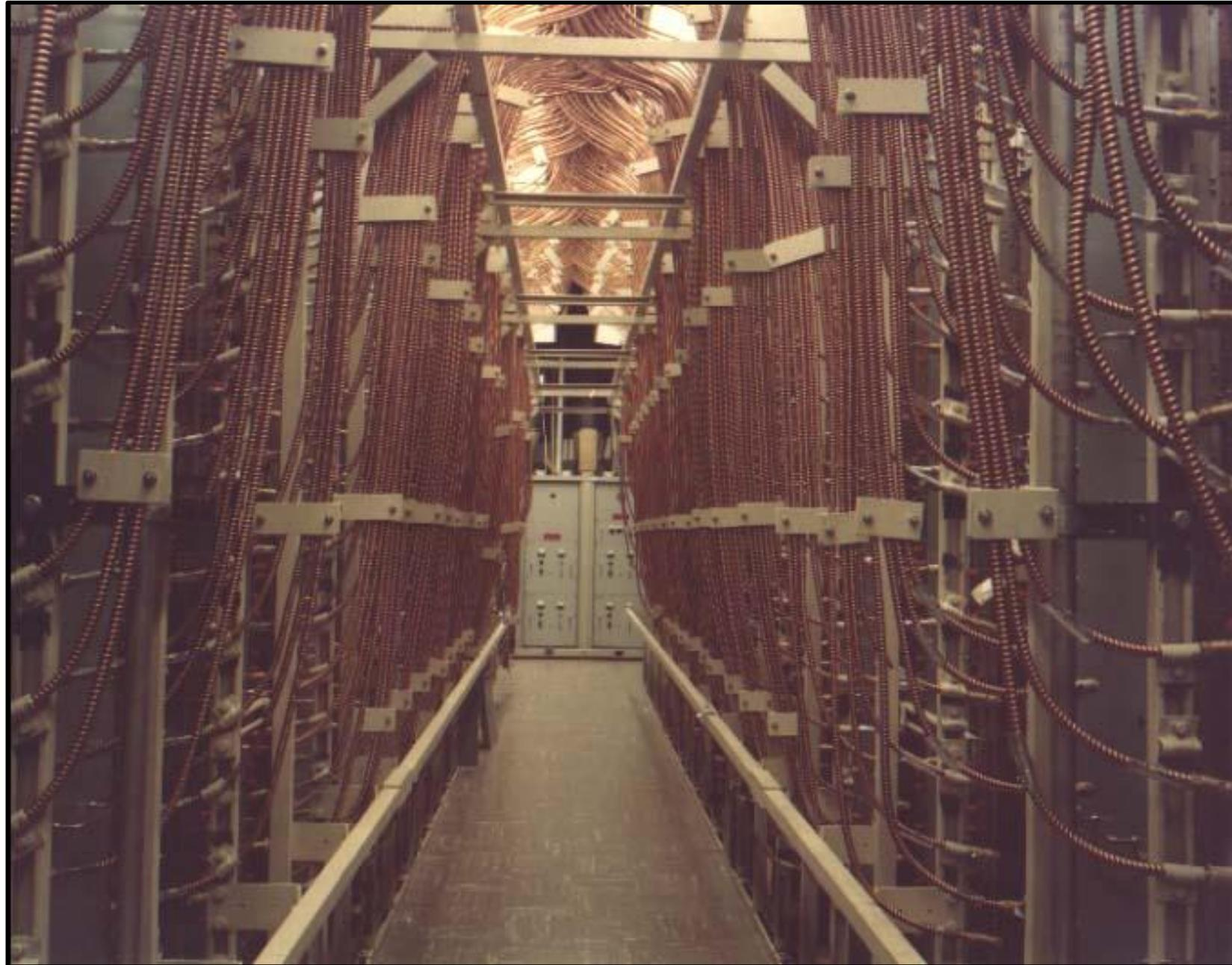
The *Beta Racks* was where the time delays were inserted to steer the beam in *Elevation*.
