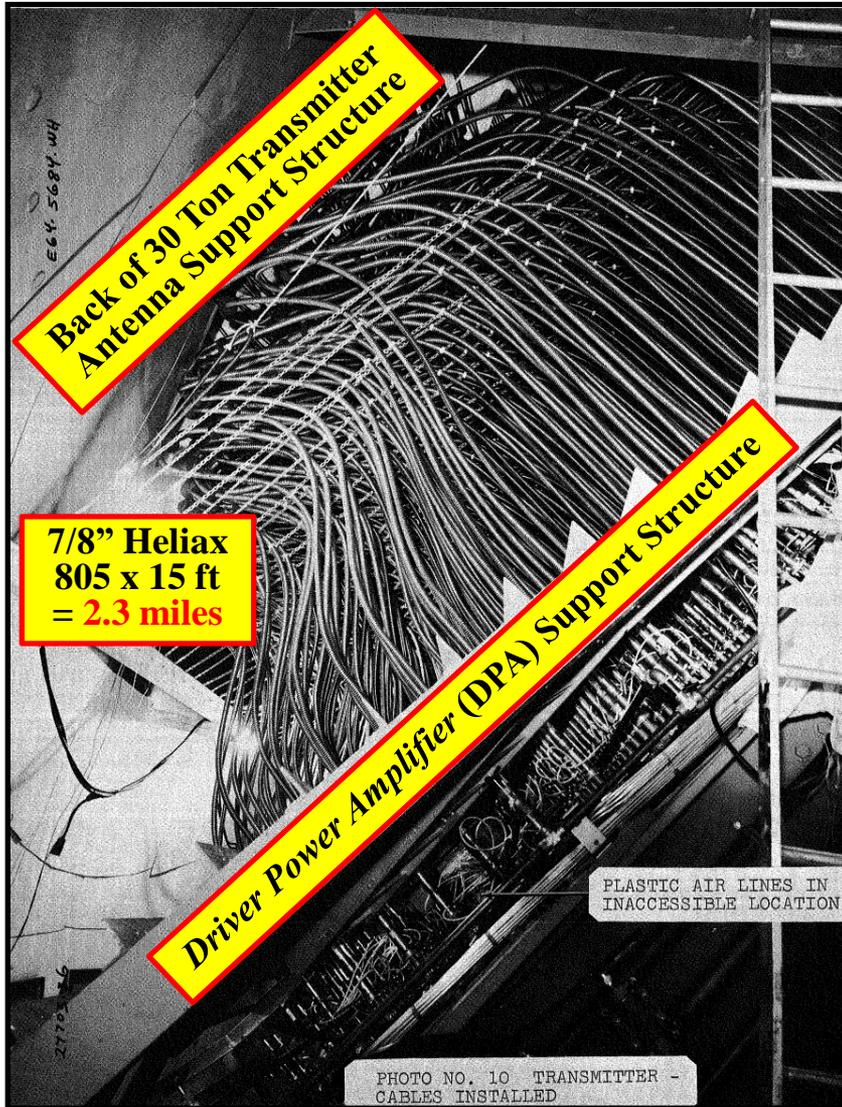
Back view of the ~900 Driver Power Amps. Note the unconnected water cooling lines.
