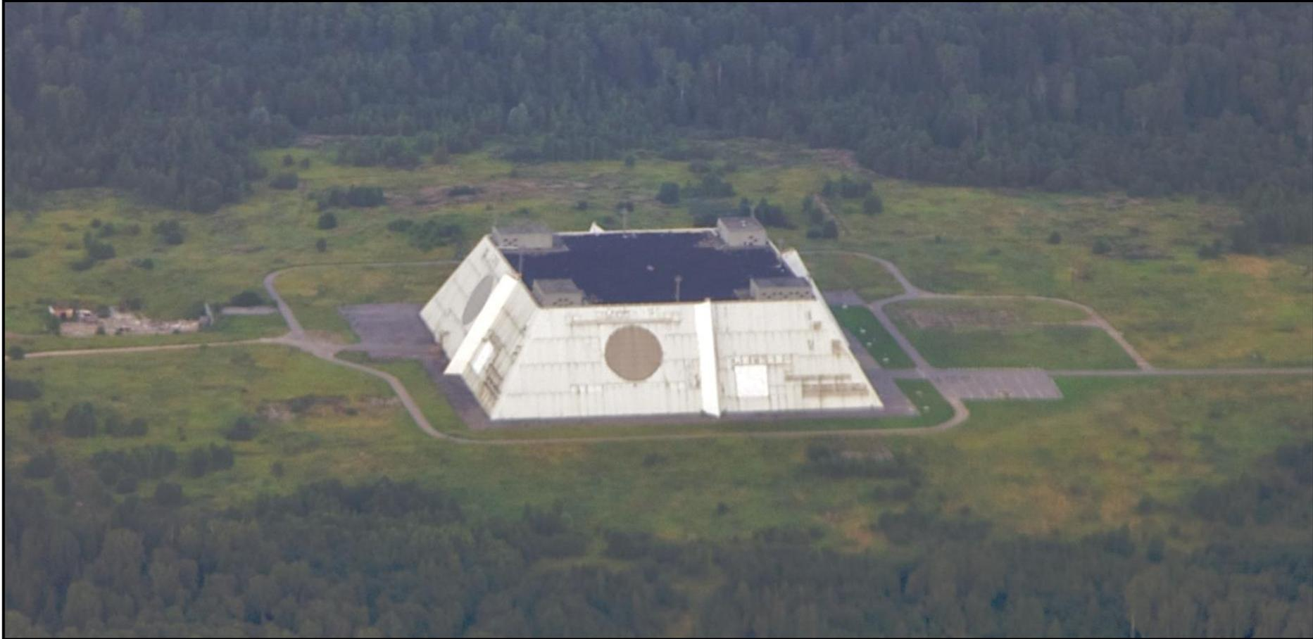
**The Soviet-era radar was developed in the period from 1973-1989. It can detect, track and discriminate ballistic targets, and guide interceptor missiles, just as the American MAR was to have done 20 years earlier.**
