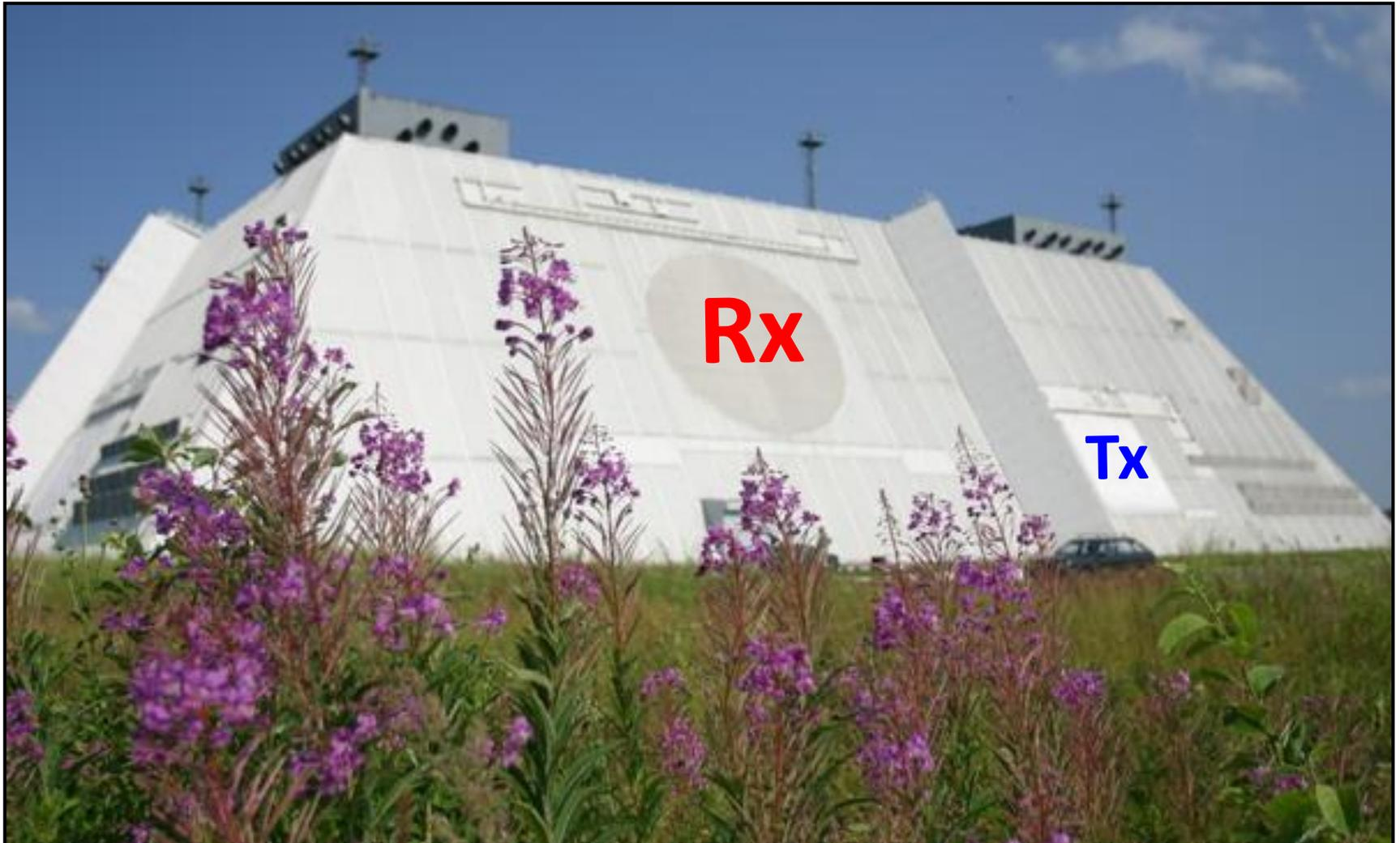
**This space-fed radar uses a circular Receiver Array 16 m (52-ft) in diameter.
