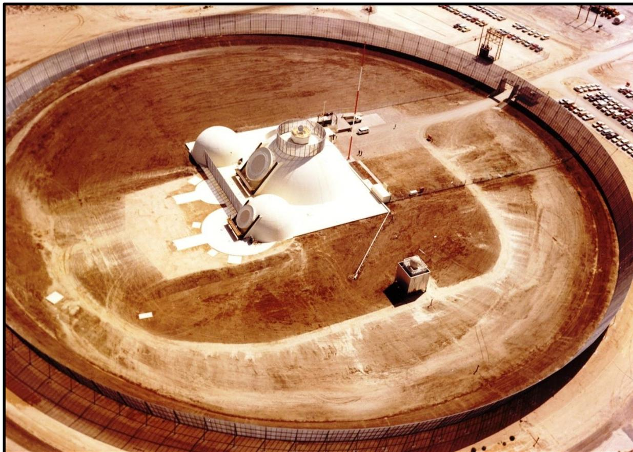
Most of the 195 x 155 ft structure is underground and extends 42 ft below surface grade.
