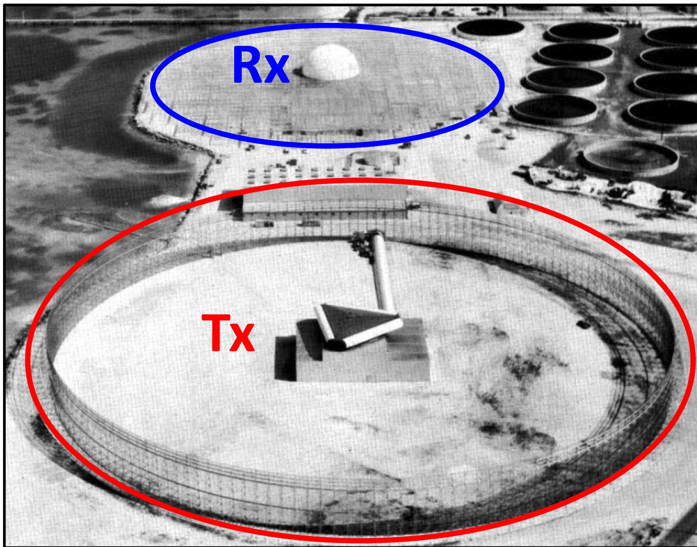
The *ZAR Transmitter* (Tx) was enclosed by a 90-ft high, 660-ft wide *Beam Forming Fence* to reduce radar “clutter” returns, and to protect staff from the high-power megawatt emissions. The triangular Tx had 3 x 80-ft long antennas which co-rotated with the ZAR Rx.
