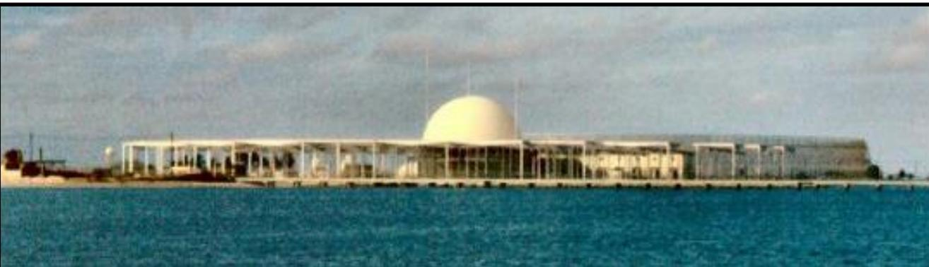
The profile view of the entire ZAR Receiver antenna showing the 120-ft white radome enclosing the 80-ft hemispherical Luneburg Lens, as well as the 600-ft diameter elevated reflecting ground plan.
