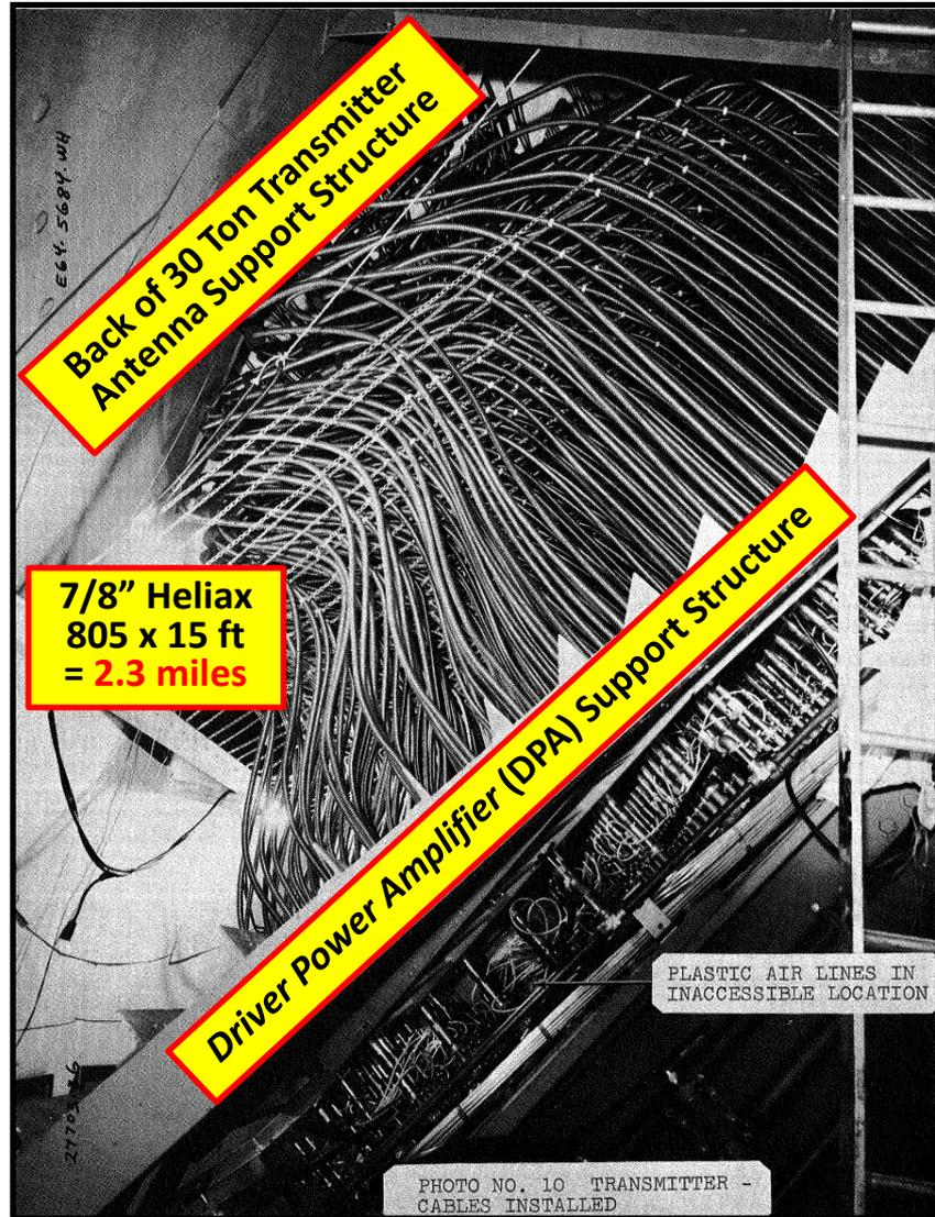
Back view of the 805 *Driver Power Amps*. Note the unconnected water cooling lines.
